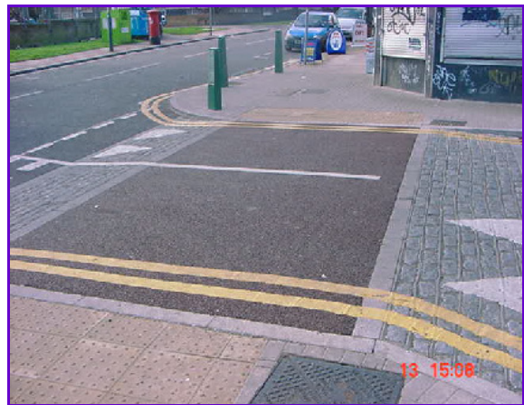
Typical raised entry treatment
